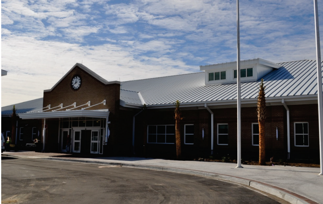
North Charleston Intermodal Center
