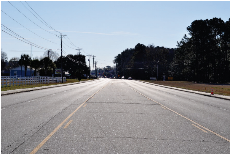
Existing conditions along US 78 looking south near Exchange Park
