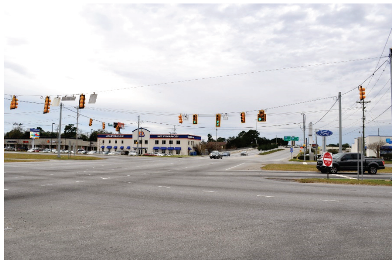
Lack of crosswalks at Rivers Ave. and Remount Rd.
