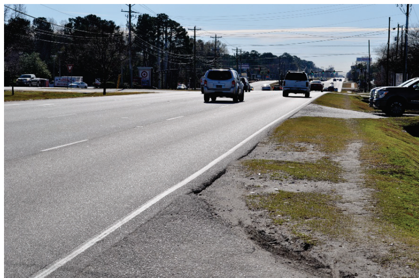
A worn path along Rivers Avenue south of Dunlap Street showing the need for pedestrian and bicycle infrastructure improvements
