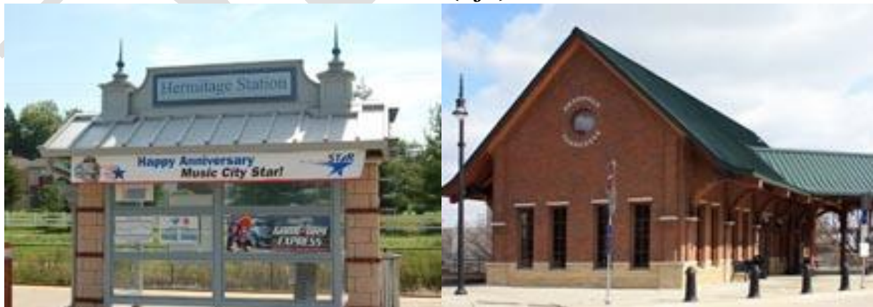
Figure 4 - 4: Hermitage Station with its simple shelter structure (left), the Riverfront station located in Downtown Nashville (right)
