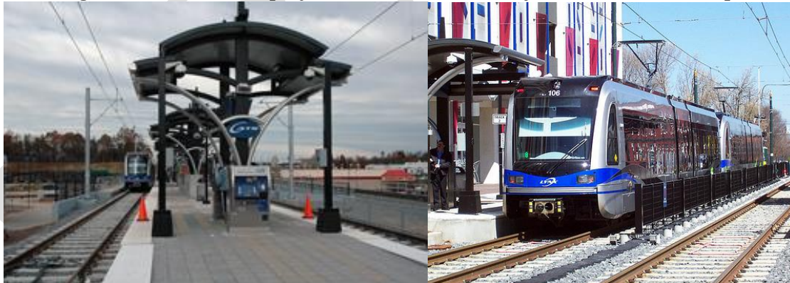
Figure 3 - 4: LYNX station platform at suburban station (left), and urban station stop
