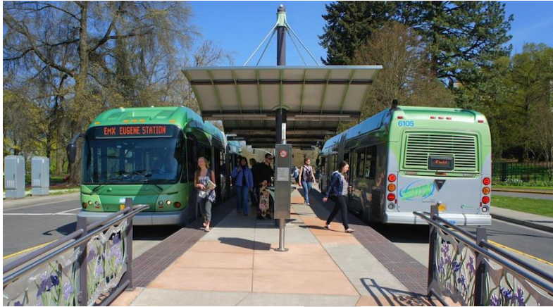
Figure 2 - 13: EmX buses serving a median station allowing left-side boarding for east and westbound vehicles.
