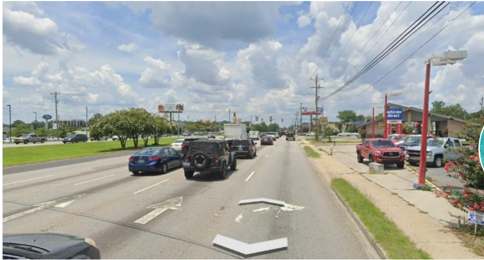
Looking north on US 78 towards station
