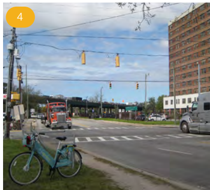
The I-26 on/off ramps near King St & Mt. Pleasant St bring high volumes of motor vehicles, including heavy truck traffic. Pedestrian facilities lack adequate width and buffers from vehicles. These streets lack dedicated bikeways.
