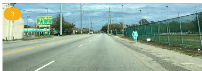
In the vicinity of this station, Rivers Ave is a 5-lane road with a center turning lane and on-street parking lanes along both curbs. Long distances between crossings encourage pedestrians and bicyclists to navigate mid-block crossings. Extra pavement could be reconfigured for protected bicycle facilities and pedestrian refuge islands.
