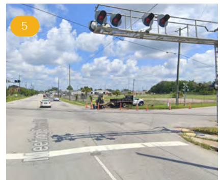
An at-grade rail crossing at the intersection of Meeting St at Milford St presents a hazard for people bicycling.
