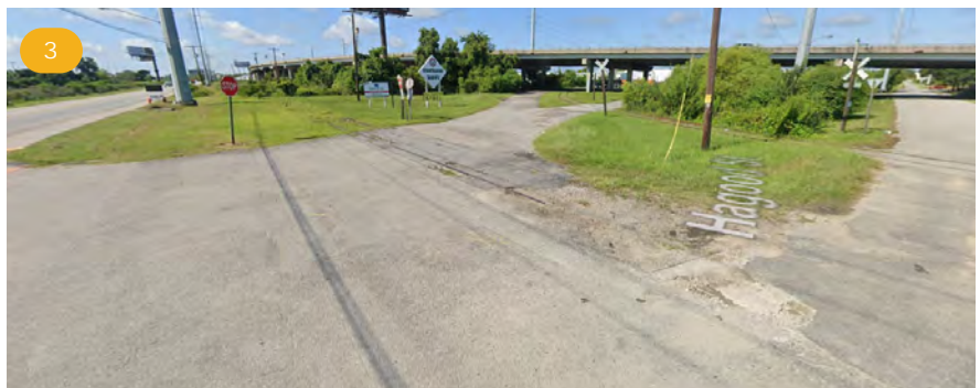
The intersection at Hagood St is very wide and lacks crosswalk markings.
