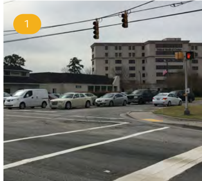
The intersection of University Blvd and Medical Plaza Dr, the access points of Charleston Southern University and Trident Health Campus, could be improved by enhancing pedestrian queuing space, incorporating high visibility crosswalks, and implementing pedestrian refuge islands.
