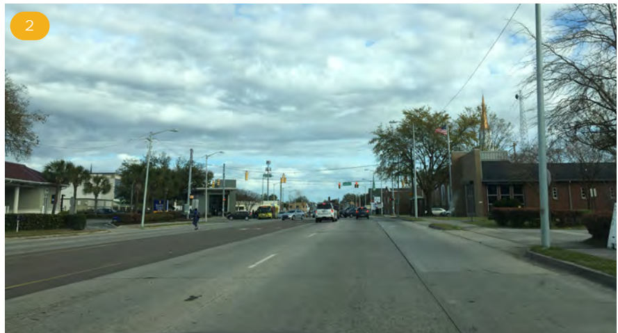
In the vicinity of this station, Rivers Ave is a 5-lane road with a center turning lane and on-street parking lanes along both curbs. Long distances between crossings encourage pedestrians and bicyclists to navigate mid-block crossings. Extra pavement could be reconfigured for protected bicycle facilities and pedestrian refuge islands.
