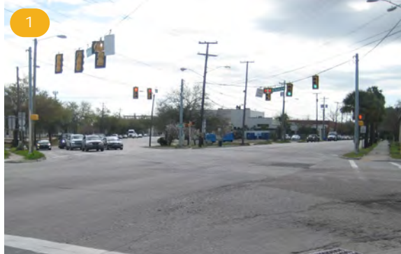
The large intersection of Meeting St /Morrison Dr /Mt. Pleasant St is challenging to navigate for active transportation users.
