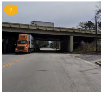
Midland Park Rd serves as an important connection for several neighborhoods and schools in the vicinity of the LCRT. The crossing underneath I-26 on Midland Park Road has potential to be transformed into a walk- and bicycle-friendly space. With two travel lanes within a 45-foot-wide right of way, there is room within the existing right of way to accommodate bicycle lanes and wider sidewalks.
