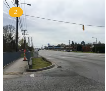
This intersection of Rivers Ave and Eagle Landing Blvd, connecting Northwoods Mall to local neighborhoods, is extremely wide and doesn't accommodate pedestrian crossings at all legs. Incorporating median refuge islands and high-visibility crosswalk markings would create a safer and more comfortable crossing.
