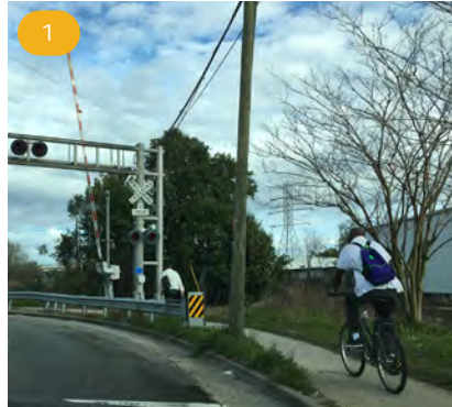
The skewed railroad crossings on Dorchester Road have high pedestrian and bicycle use. South of the rail crossing, there is a significant sidewalk gap on one side with evidence of people walking in the grass.
